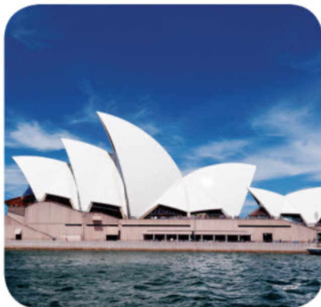
The Sydney Opera House Australia
